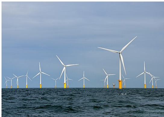
Belwind offshore wind farm on Bligh Bank in the Belgian North Sea, 2 October 2012. © Hans Hillewaert / Wikimedia Commons · CC BY-SA 4.0
